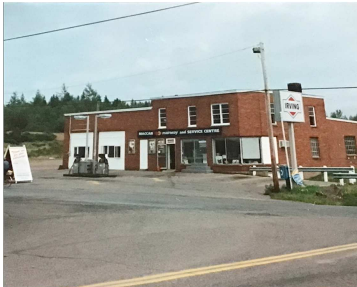
Maccan Garage (Picture taken just before it was demolished)
